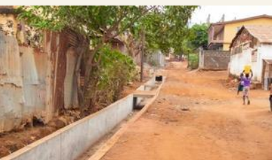
Constructed over 2.2 km of drainage in 11 communities
