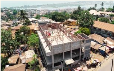
Entered final stage of Wilberforce market construction
