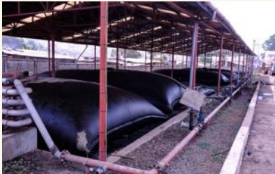
Built and operationalised Freetown's first Wastewater Treatment Plant
