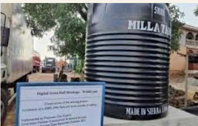
Installed 160 water storage tanks & rain harvesting system in communities & PHUs
