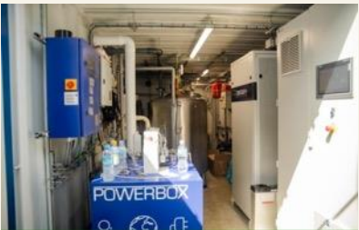
Installed a biogas plant at Mabella Market
