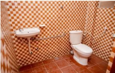
Installed 10 biodigester toilets at Susan's Bay
