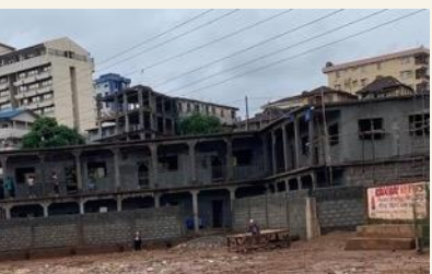
Commenced construction of 12 classroom primary school in Kroo Bay community
