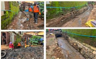
Conducted extensive flood mitigation activities before the rainy season
